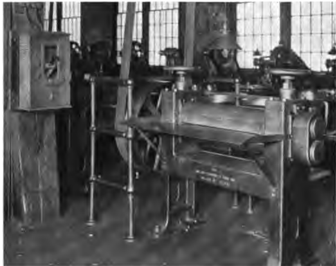
Fig. 5. Protected Flattening Rolls.†
